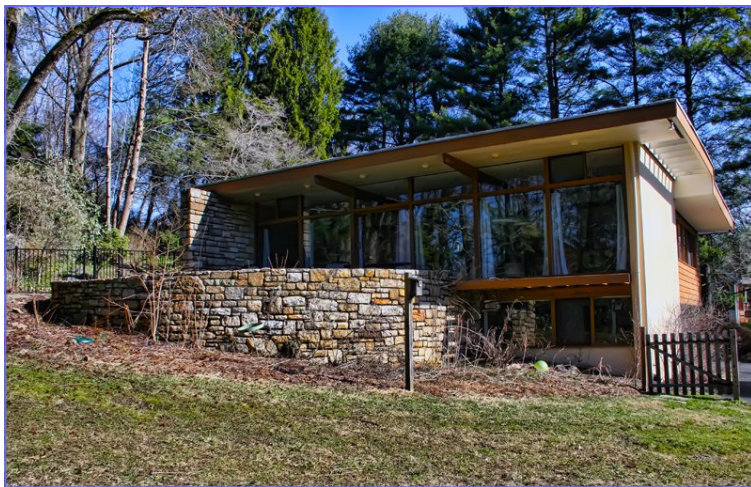
The Zapruskis Residence in Thornbury, Pennsylvania (architect Rudolph Zapruskis).
