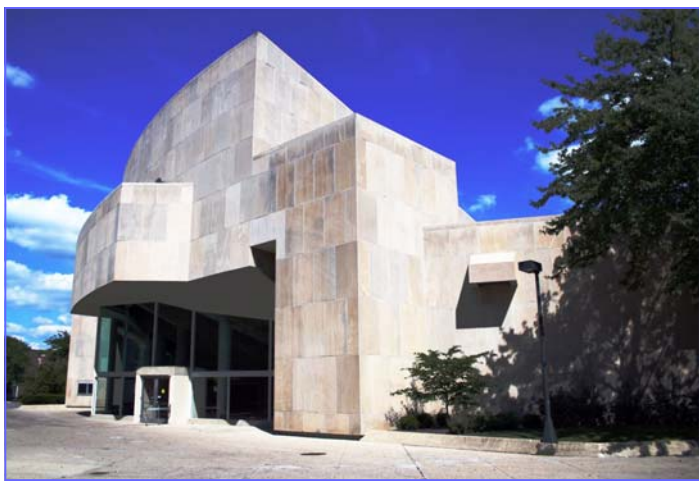
Pruis Hall at Ball State University in Muncie, Indiana (architects Evans Woollen and Associates).
